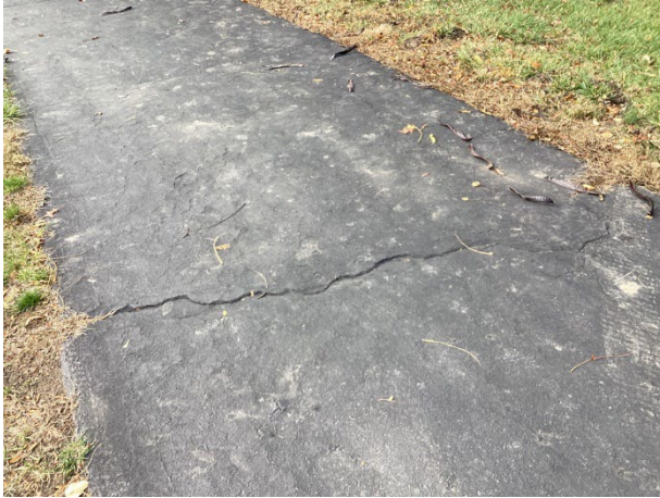
Pavement cracks
