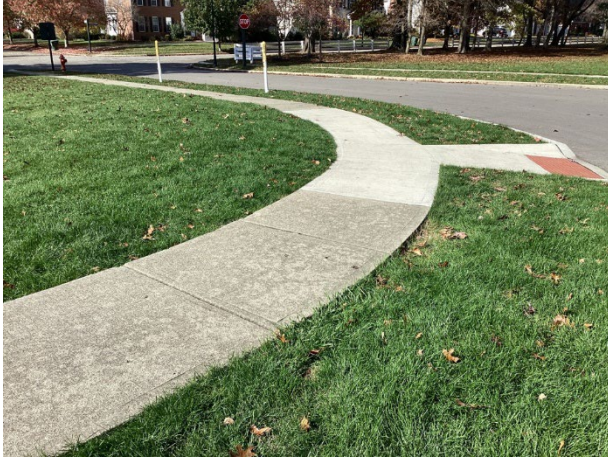
Concrete sidewalk overview
