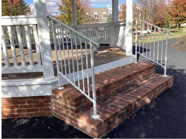
Masonry steps and metal railings
