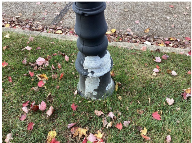
Finish deterioration
