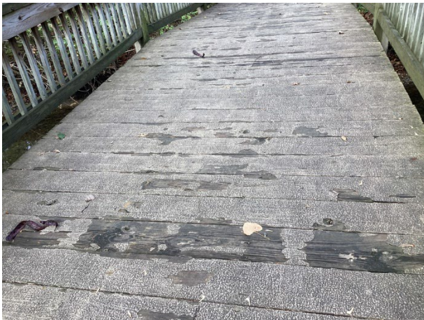
Surface deterioration
