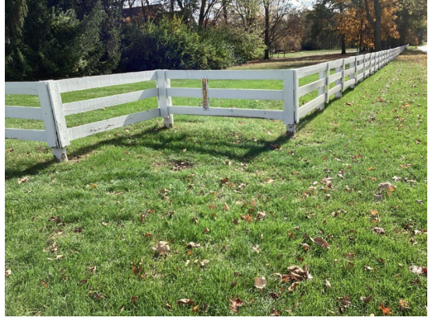
Wood fence overview
