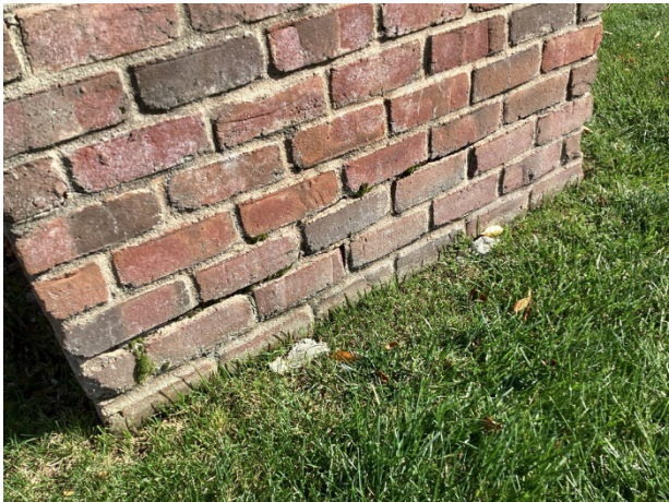
Mortar loss at Fernridge Dr
