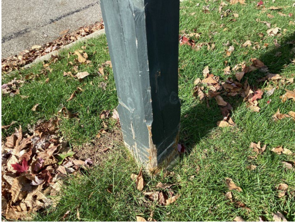
Finish deterioration
