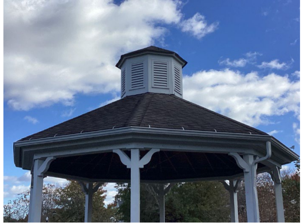
Asphalt shingle roof
