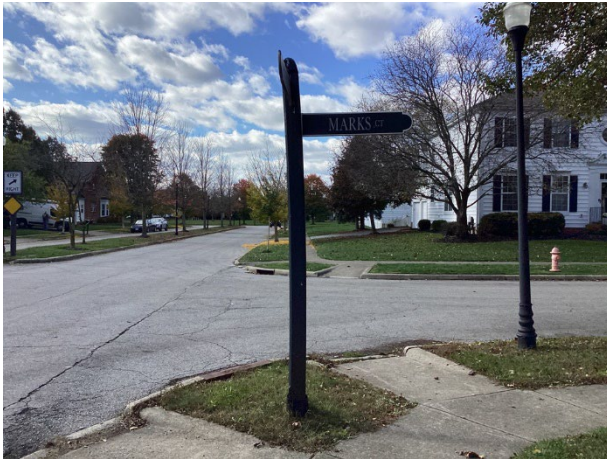
Warped wood post
