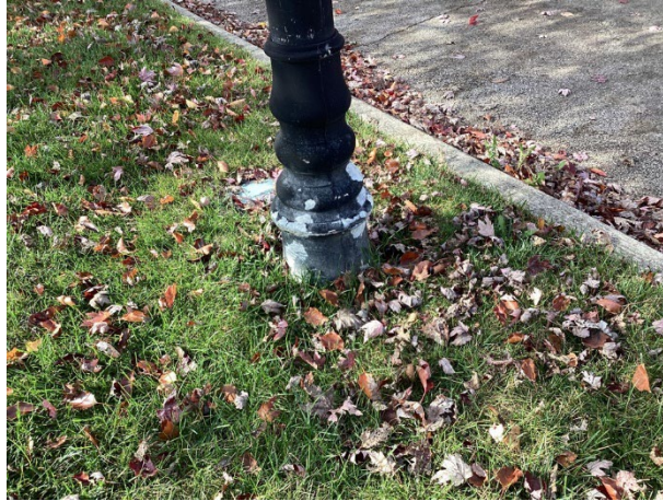
Finish deterioration
