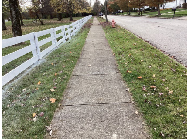
Concrete sidewalk overview
