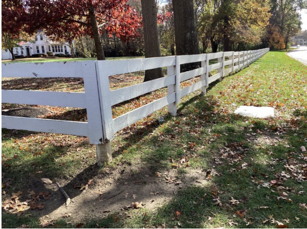
Wood fence overview
