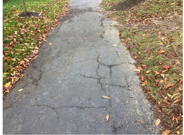
Settlement cracks
