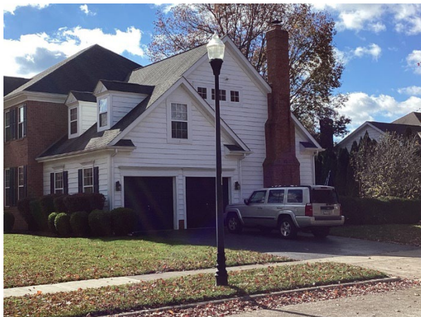
Light pole and fixture
